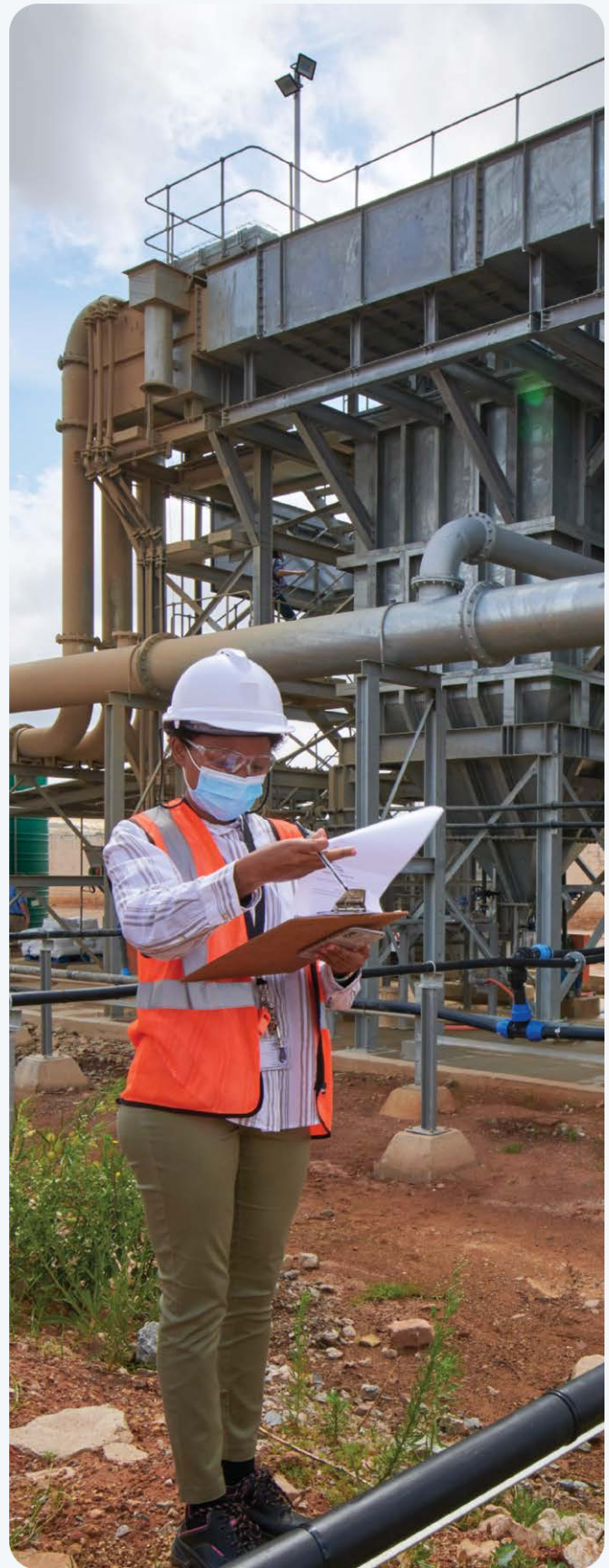
Water treatment plant at the Cooke operation, SA gold operations
