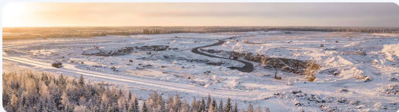
Syväjärvi open pit mine site, Keliber lithium project, EU operations
