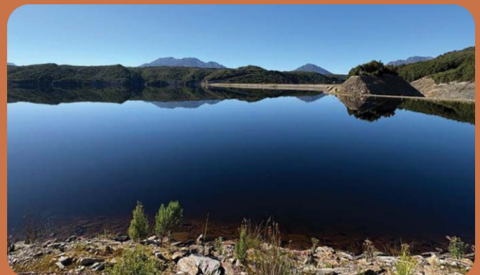
Princess Creek tailings storage facility at the Mount Lyell copper project, AUS operations
