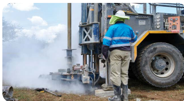
Water borehole drilling at the SA PGM operations
