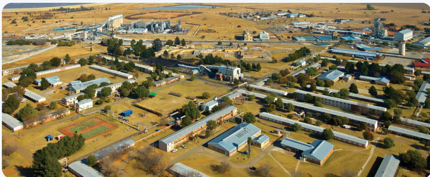
Infrastructure at the Beatrix operation, SA gold operations
