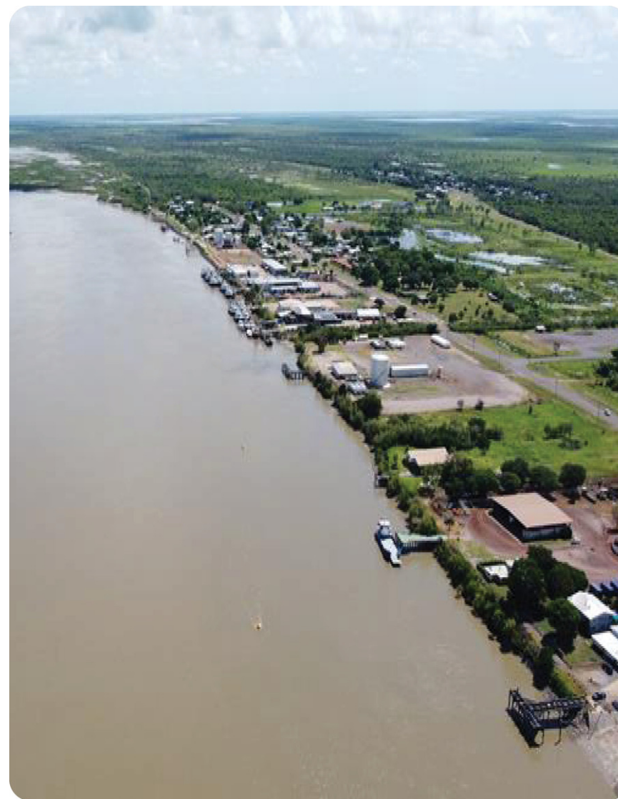
Karumba port facility, Century zinc tailings retreatment operation, Queensland, Australia
