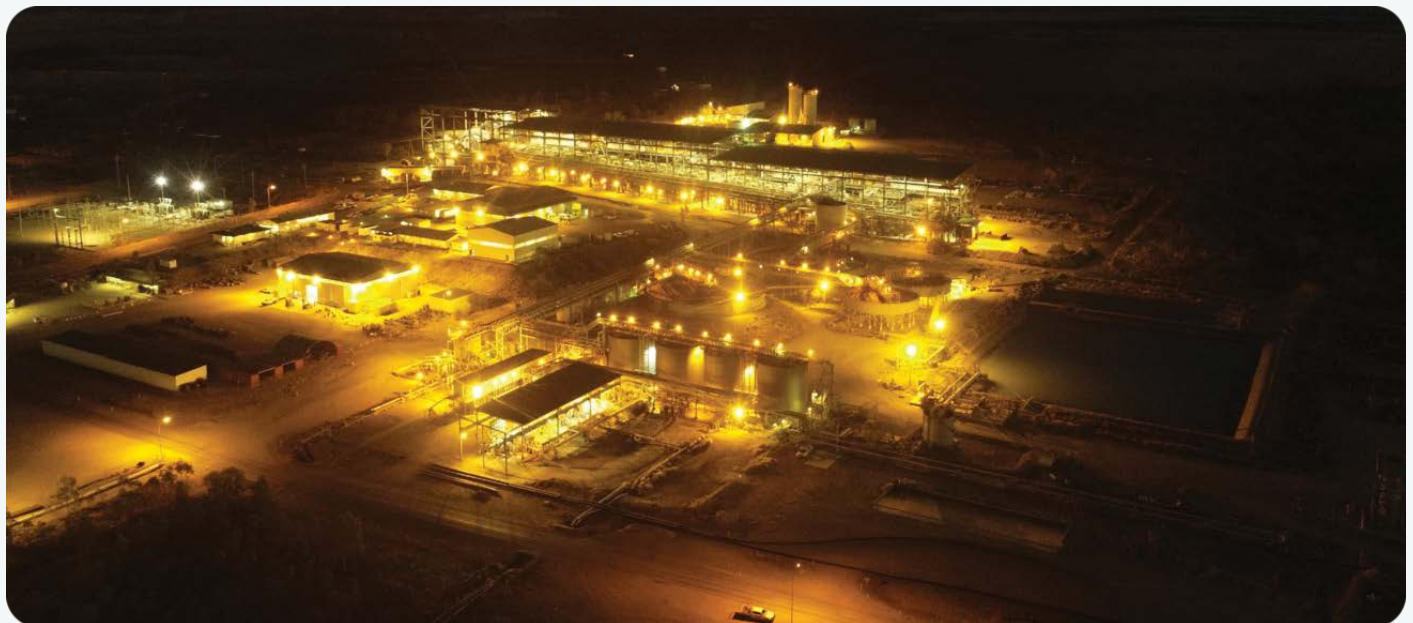
Processing plant at the Century operation, Australia
